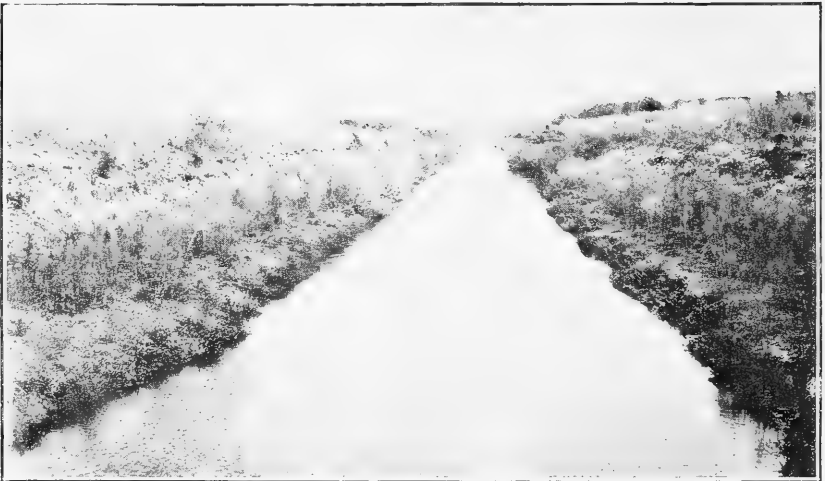
FIG. 2.—COURSE OF MAIN DREDGED CHANNEL, NEAR FELLSMERE, FLA., ADJOINING SLOPE COURSE. THIS VIEW REPRESENTS FAIRLY WELL THE CONDITION OF THE CHANNEL ALONG THE SLOPE COURSE. 1917. (SEE TABLE NO. 6.)
